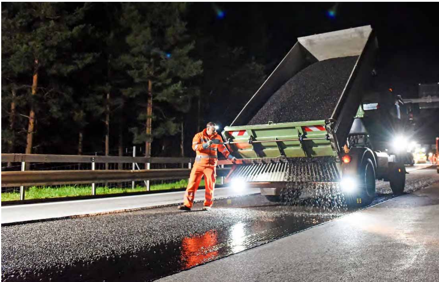
Applikation der SAMI (Stress Absorbing Membrane Interlayer)
