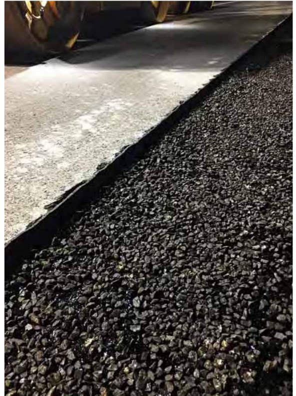
Applikation der SAMI (Stress Absorbing Membrane Interlayer)
